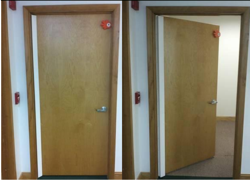
Finger Shielded -Push Side Door (framed on left) Door Closed and Open View
